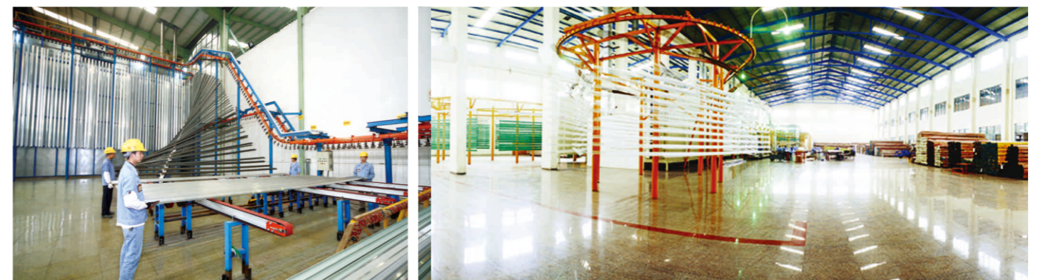
氟碳喷漆车间 PVDF Painting Plant
